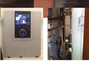
thermal panels, the wood burner or the oil fired boiler. By having a cylinder with three coils it means that each of the three heat sources can be programmed to heat the hot water independently. The oil fired boiler will only heat the water when the solar thermal and wood-burner have failed to do so.
